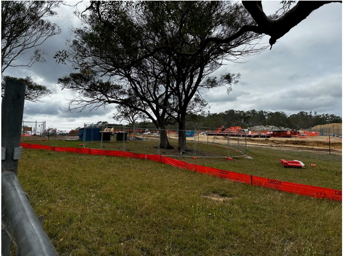
Photo 1: Tree Protection Zone fencing
