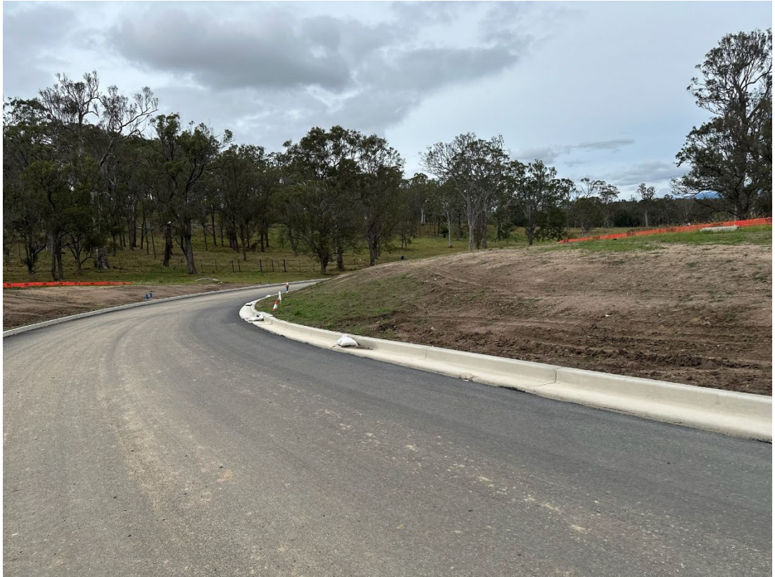
Photo 5: Internal road construction and batter stabilisation
