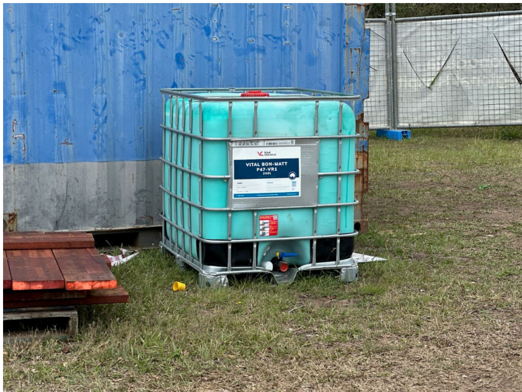
Photo 8: Chemical dust suppression bonding agent
